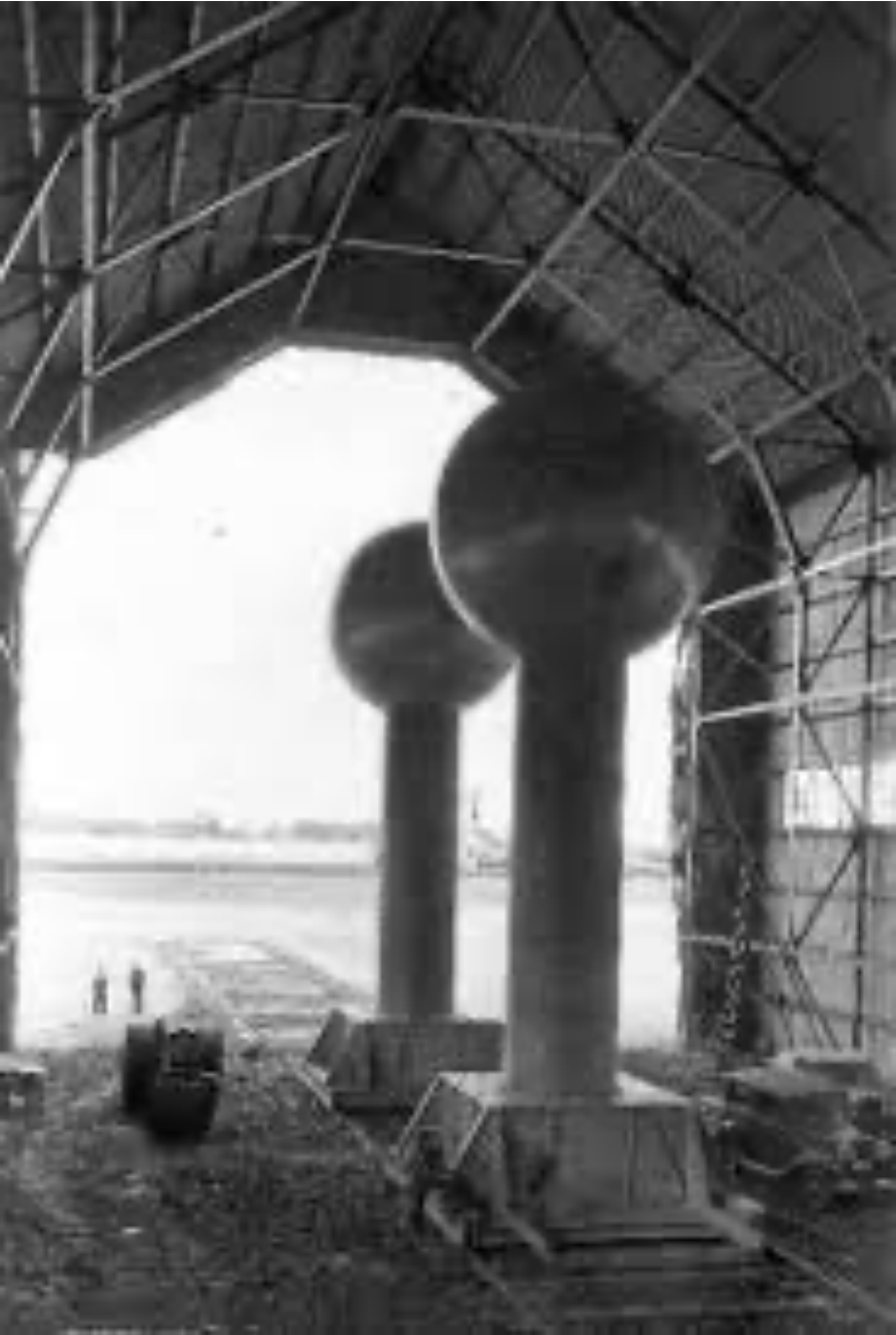
Van de Graaff's very large accelerator built at MIT's Round Hill Experiment Station in the early 1930s. 43feet above the ground.
