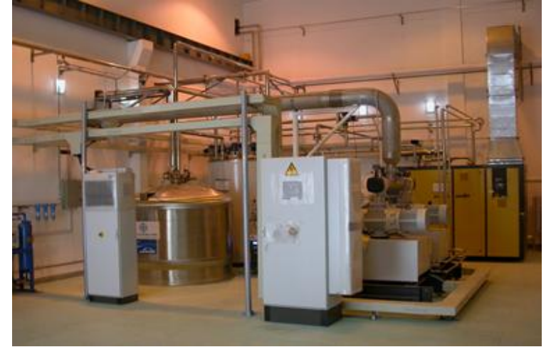
Large-scale 2 K Cryogenic Circulating Liquid Helium System
