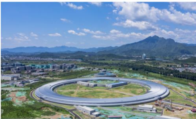
Figure 1: The HEPS building complex. The circular storage ring is 1360.4 m. The extension buildings from this ring reflect its magnifier design.
