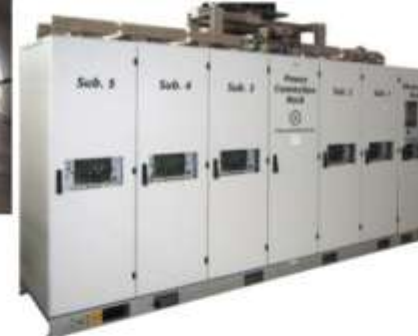
LHC 13kA power converter
